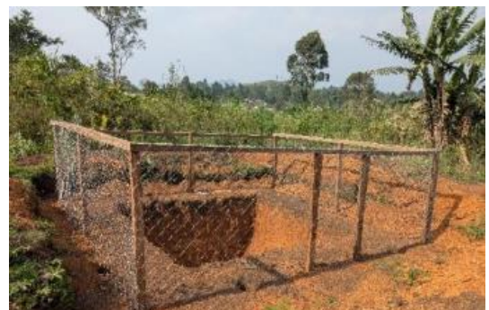
Waste pit at the Bale health facility. ©Medair
